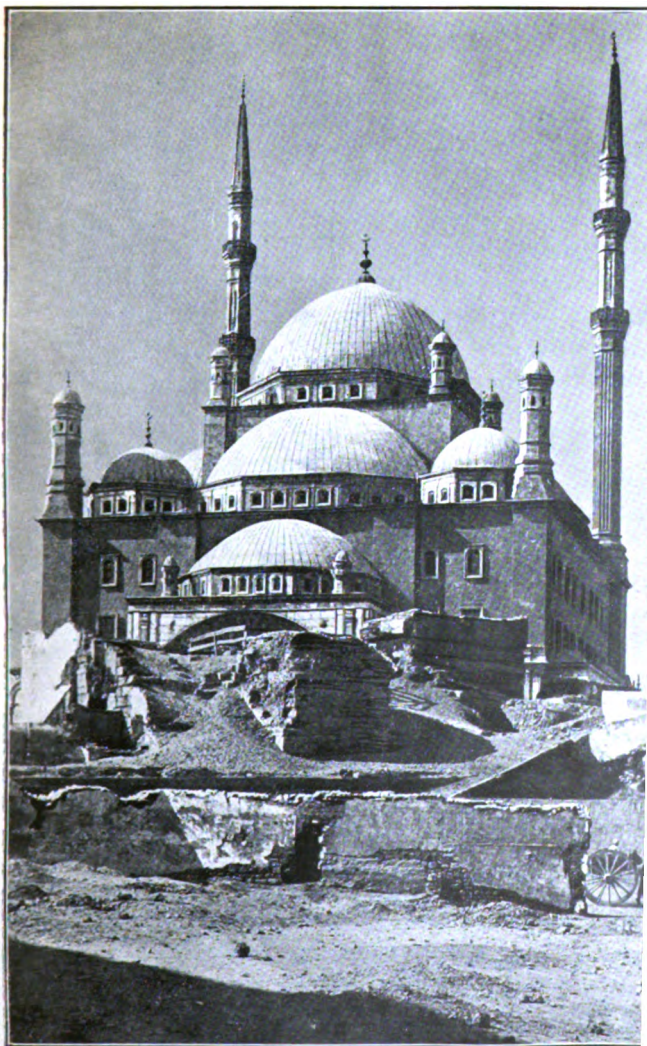
PLATE 14.—A Mosque at Cairo, showing the four corner minarets and the central cluster of five domes.
